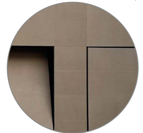
Particolare porta filo muro Detail of the door flush with the wall
