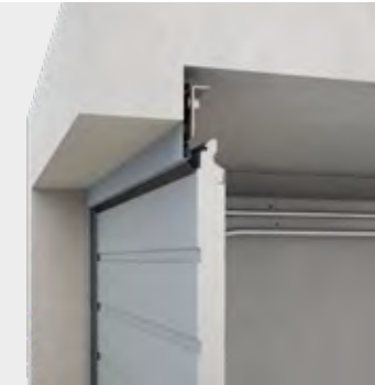
Behind The Lintel
